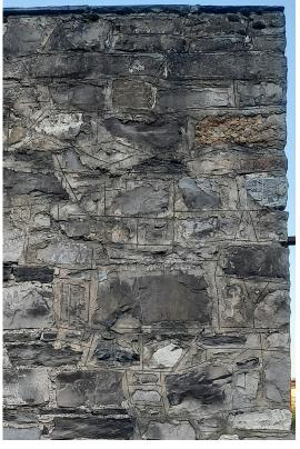
Fig. 4.2.16 - Section of rebuilt masonry with cementitous mortar
