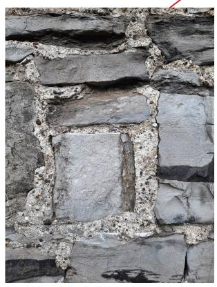
Fig. 4.2.15 - Typical lime mortar found along lower section of wall
