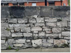
**Fig. 4.2.30** - Concrete blocks replacement at upper section
