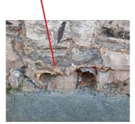
Fig. 4.2.23 - Loose masonry at Fig. 4.2.24 - Clay pipe outlets lower section
