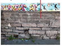
**Fig. 4.2.22** - Concrete blocks replacement at upper section. Pointing washed out at lower section and loss of a few facing stones
