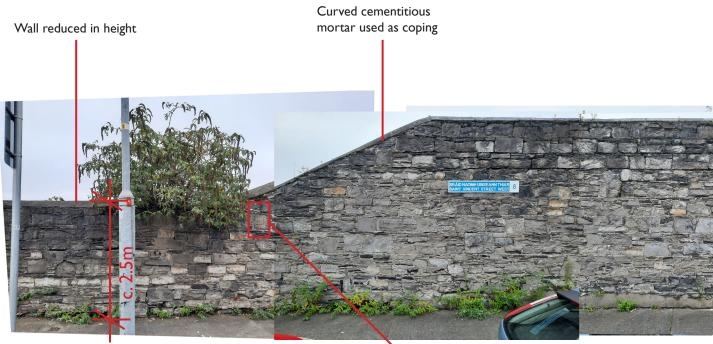
Fig. 4.2.12 Existing Boundary Wall Elevation A - St.Vincent's Street West
