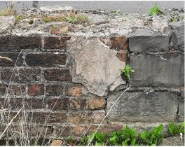
**Fig. 4.2.27 -** Modern section rebuilt with concrete blocks
